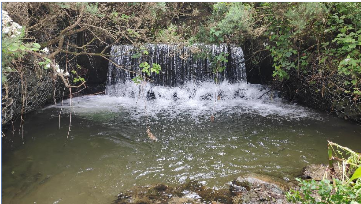
Plate 4.1 The weir at site A13 on the Kilbane Stream was a significant barrier to fish
